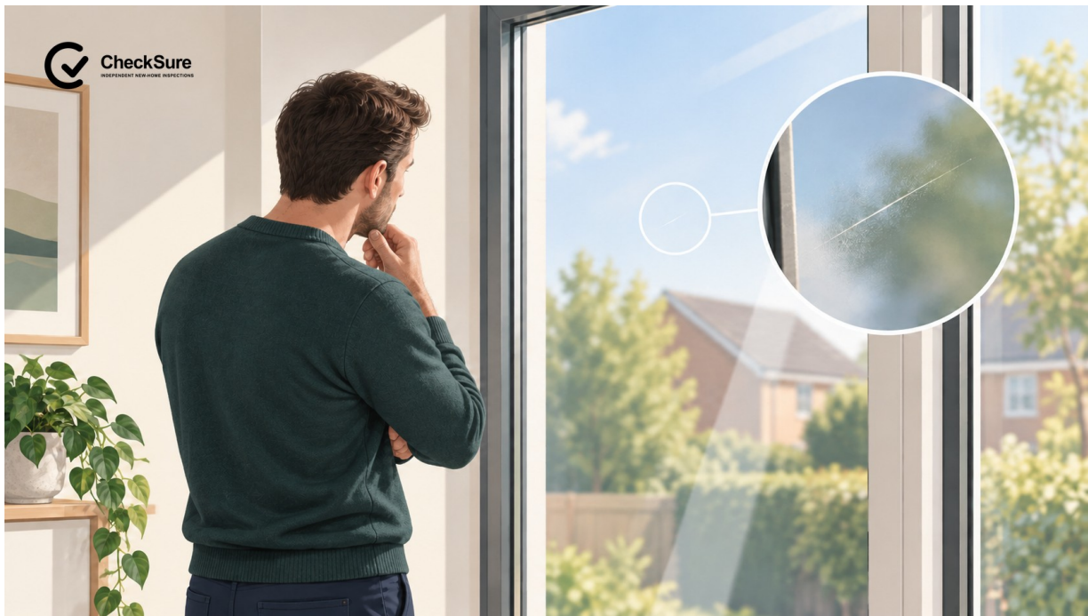
Figure 1. Inspect clean glazing in normal daylight from the specified viewing distance before deciding whether a mark is unacceptable.
