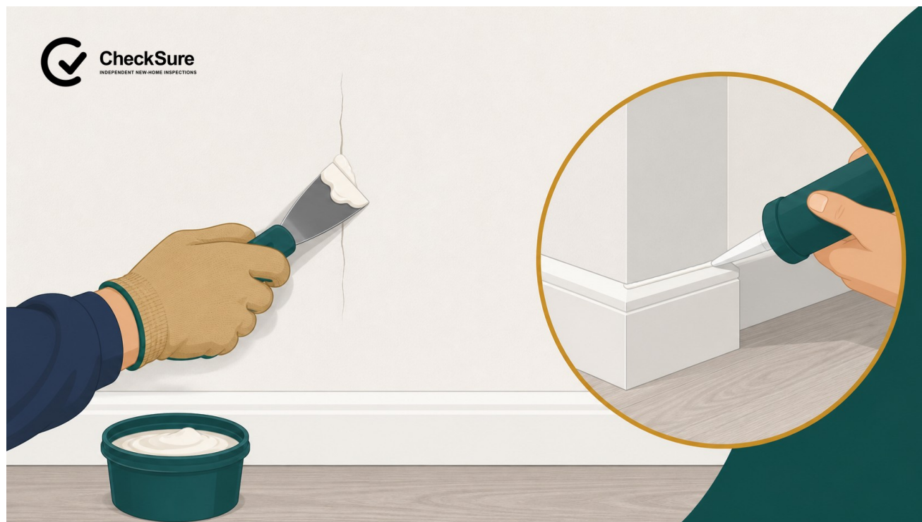
Figure 1. Small, stable cracks within plaster and at material junctions need different repair products; investigate warning signs before decorating.
