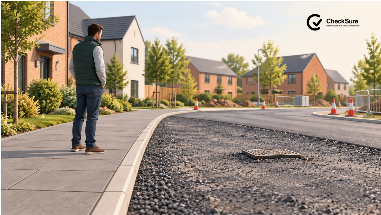
Figure 1. Estate roads may remain unfinished during construction, but access routes and pavements should still be safe and usable.
